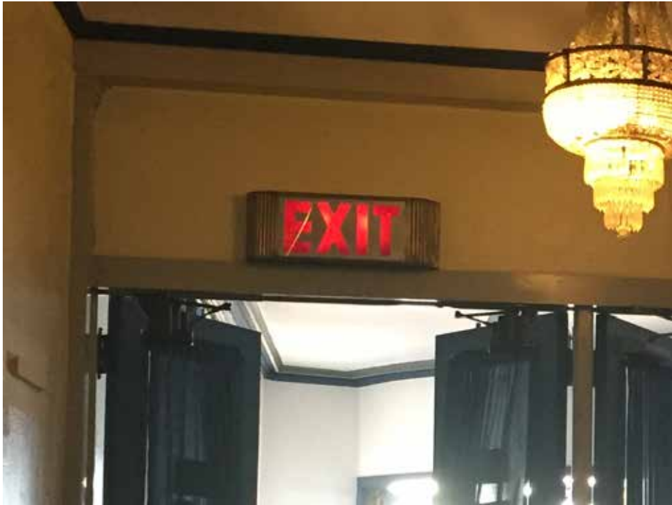
(Typical Pre-Restoration Photograph)
