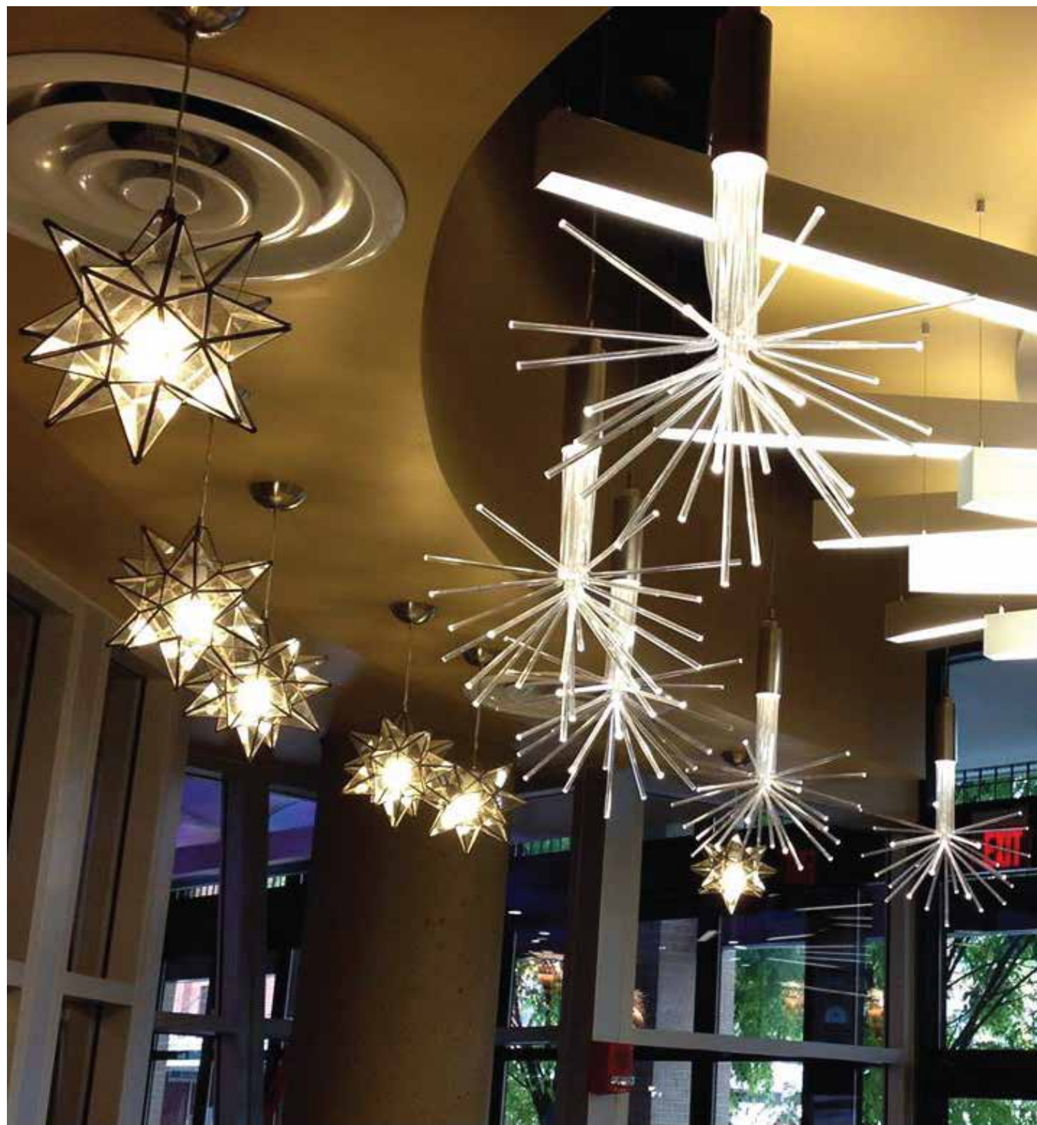
Custom Fabricated Light Fixtures Installed On-Site
