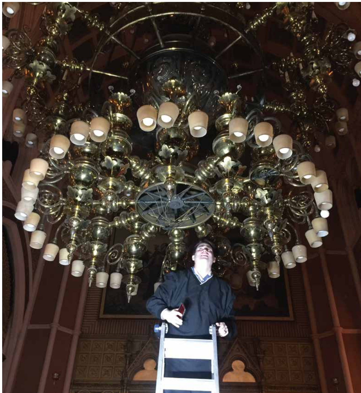
On-Site Electrical Inspection of Grand Chandelier
